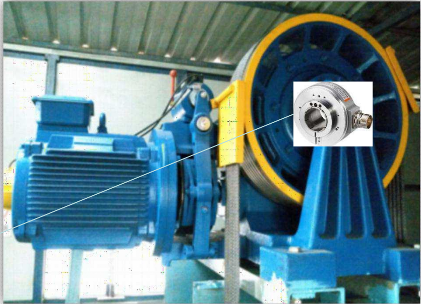
MOTOR ENGRENADO (GEARED) / ASSÍNCRONAO COM ENCODER
